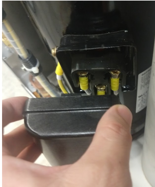
Figure 6: Remove black cover and 4 screw terminals
