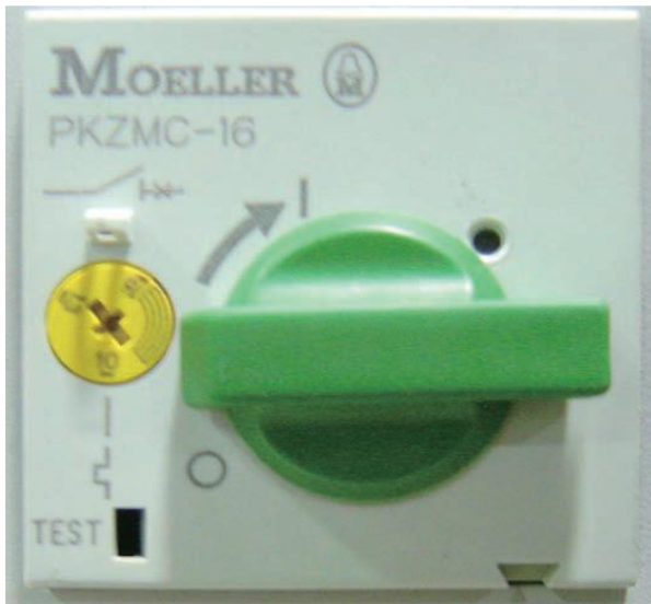
Figure 9 Main Power Switch
