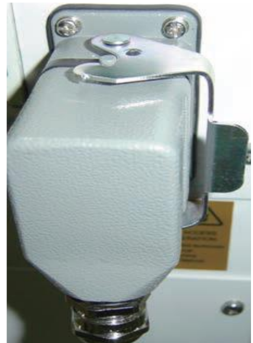
Figure 8 Connect mains power supply cable to mains power receptacle
