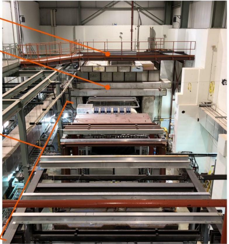
NM4: looking upstream
